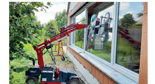
Suitable for outdoor use to move windows from the outside to the inside
